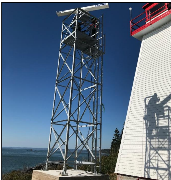
Figure 6: One of two high-resolution radars constructed near the FORCE site to be used for the RAP program.
